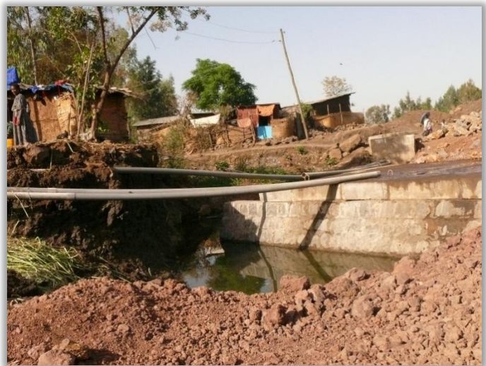
Figure V.A: Neighbourhood Next to the Road Construction – Kebele
