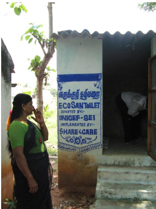
Image 1.1, example of an ecosan toilet in the rural area of Tamil Nadu
