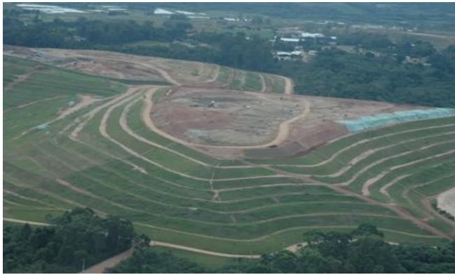
Pic.3.1 - An aerial photo of the sanitary landfill of Caximba .
