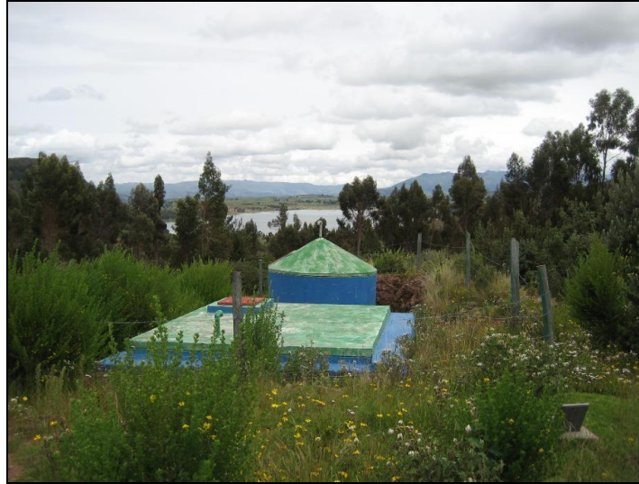
Picture 3: Reservoir found in Taucca used for drinking water (M. Verkooijen)
