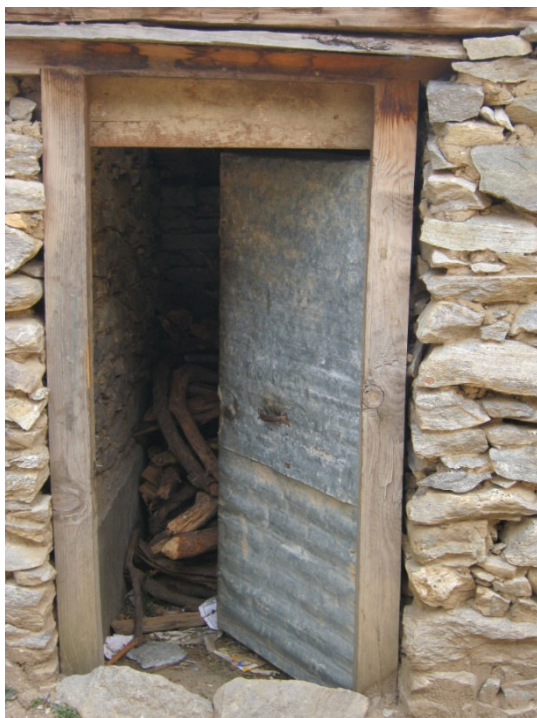
Picture 2 Wood storage in sanitary facility
