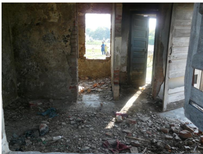
Figure 11 Inside the sub-centre at village V
