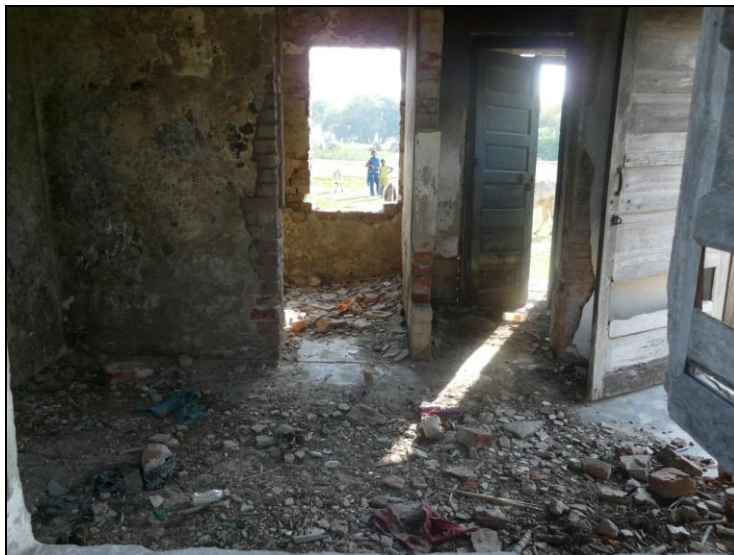
Figure 8.4 View inside the sub-centre (photo taken by the student)
