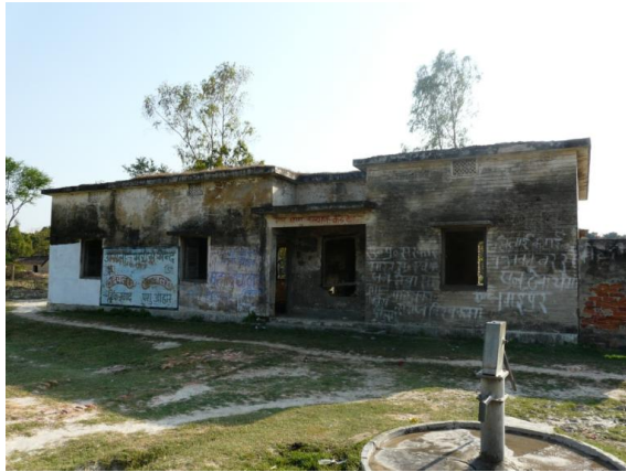
Figure 10 Sub-centre in village V
