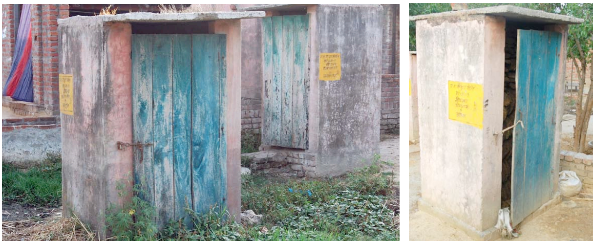
Figure 7.10: Common TSC Latrines in Kaundada 37
