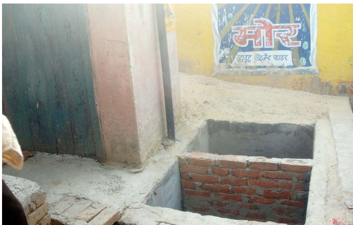
Figure 7.12: Newly Constructed Pucca Substructure in Kaundada
