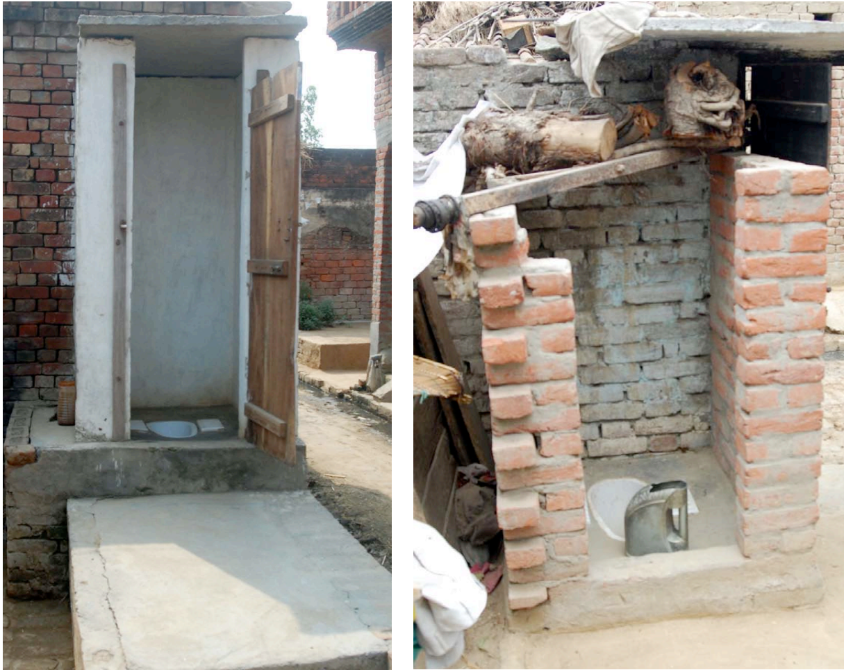
Figure 7.13: Common TSC Latrines in Simra Keshopur
