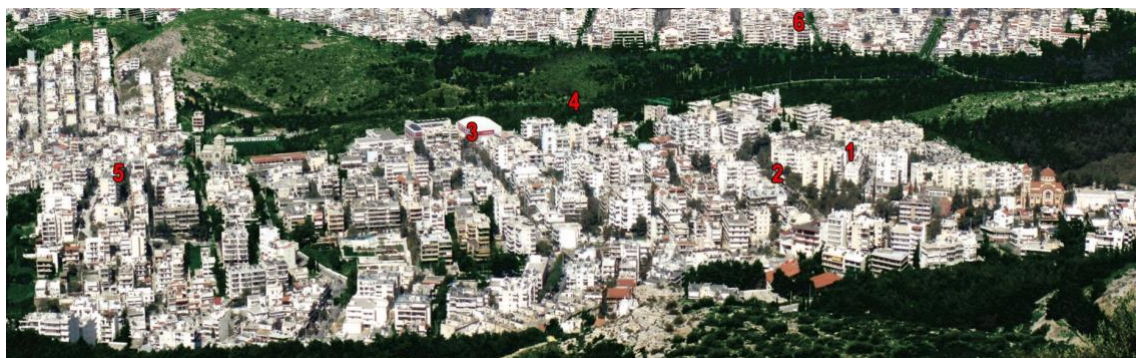
Pic. 5.1-3 Kareas district, view from mount Hymettus. 1) Social housing complex, 2) central road, 3) elementary and high school, 4) Hymettus peripheral Motorway A64, 5) borders with the municipality of Ilioupoli, 6) Vyronas municipality
