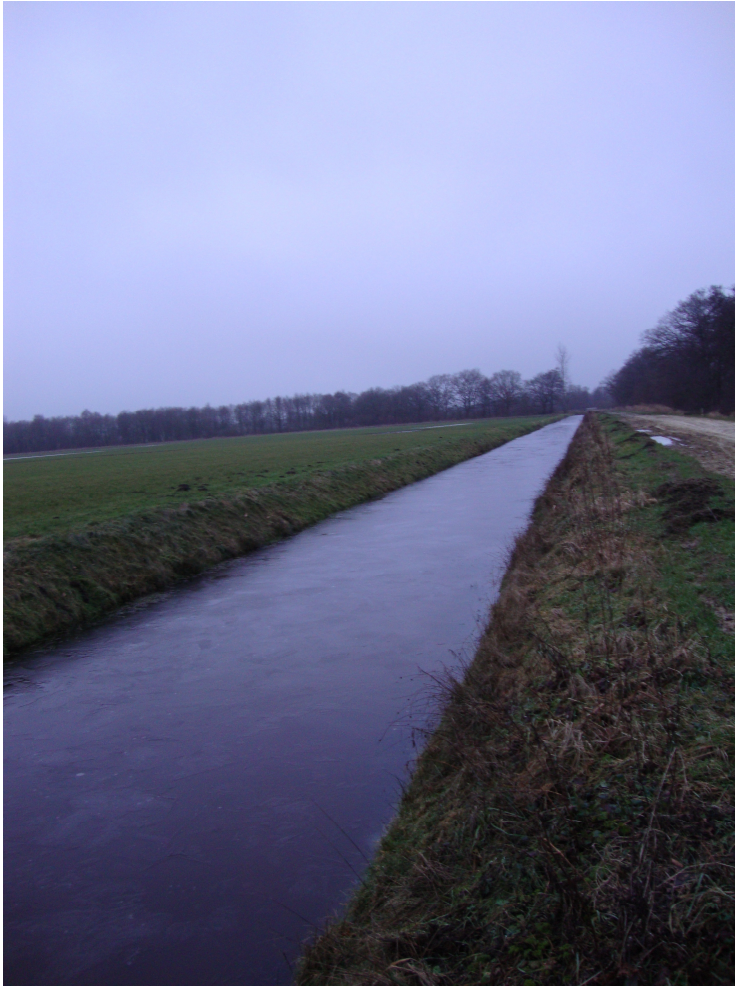
Figuur 27 Waterway of class 3 on the flank of the Elperstroom
