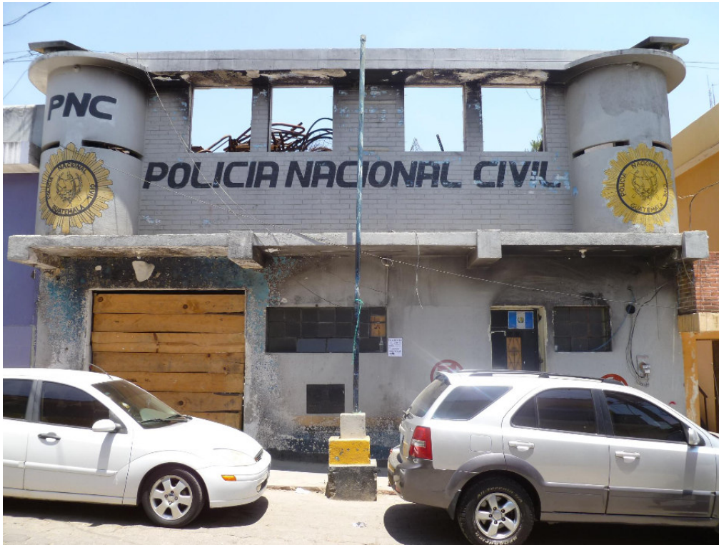
Photo 3 shows the police office in Sololá that was damaged after a lynching that took place in November 2009. Citizens of Sololá set the police office on fire to get a hold on three people that were suspected of killing a bus driver and a passenger in a bus in Sololá. The police office is still not repaired.
