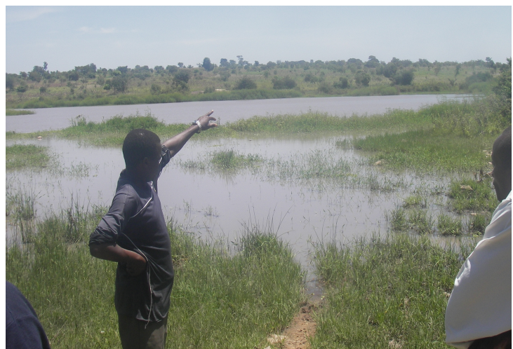
Figure A: Buzilasoga Dam, Sengerema District, constructed in colonial times.
