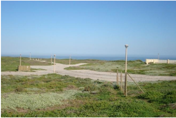
Photo 5.2: Empty plots with infrastructure
