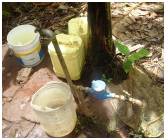
Image 4-1. New water meters
