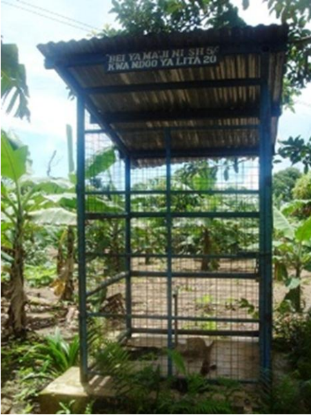
Image 4-2. Abandoned water kiosk
