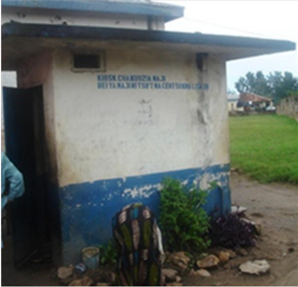
Image 4-4. Water kiosk built by BUWASA
