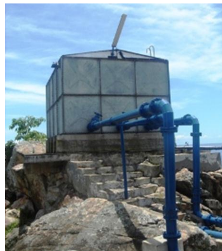
Image 3-2. Water infrastructure built under LVWATSAN
