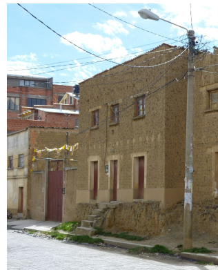
Image 3.1: Typical building in the Zona 16 de Julio
