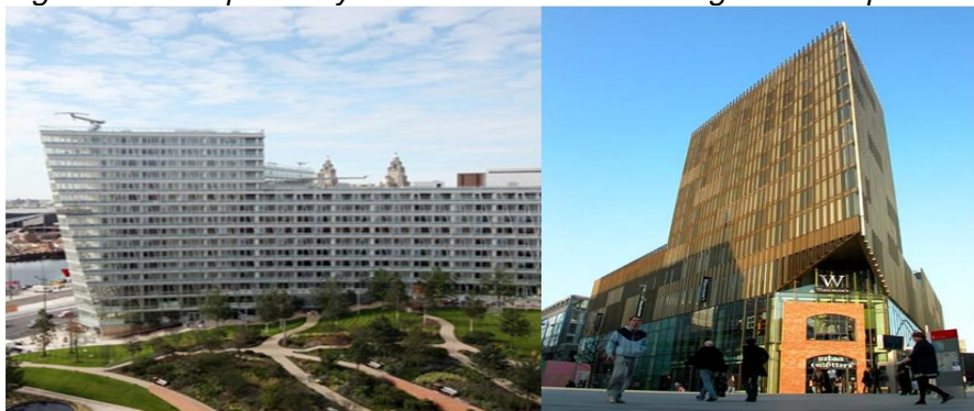
Figure 3.3: Respectively One Park West and Bridge Street apartments in Liverpool ONE
