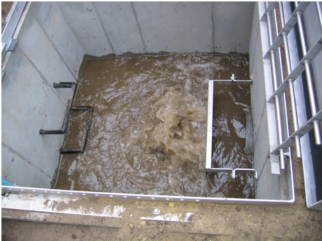
Figure 4 – A deep infiltration well 'burping' with the trapped air. The inlet of storm water is to the right. Photo Copyright IF-technology, Arnhem, The Netherlands.
