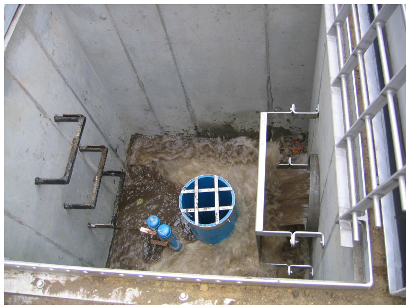
Figure 9 - The large diameter well in its construction basin. A screen is present to divert the flow from the adjoining pipeline
