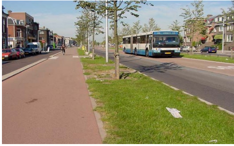
Fig8: the high-quality public transport lane on the "Vleutenseweg". One of the sections of the bus lane network that has already been realised. From left to right the photo shows a parallelroad, a bicycle path, a grass verge, the main road, the bus lane and the central reservation of the road.
