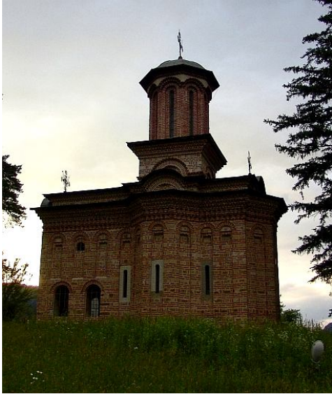
Figure 5.1. The Hospital Church from Cozia
