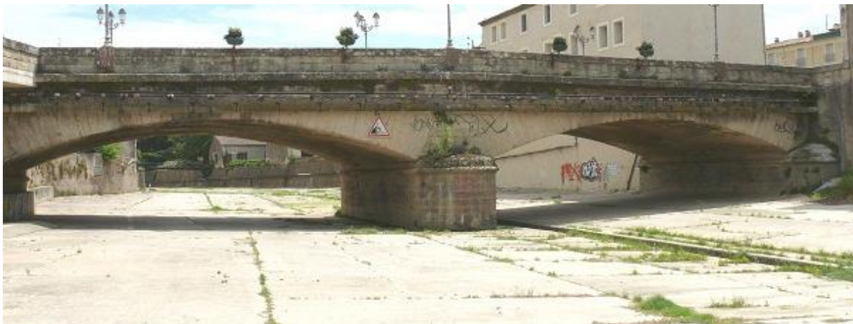
Figure 5.3: Pont du Peyne crossing the concrete floodplain in Pézenas (Janberg, 2010)
