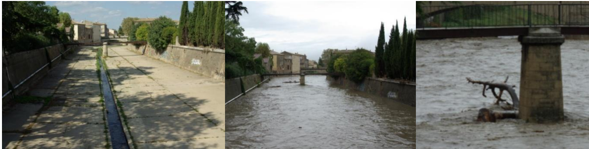
Figure 5.2: a) The concrete floodplain with the Peyne centered in a 25cm wide ditch under normal conditions (18 September 2009); b) The concrete floodplain during a minor flash flood (21 st October 2009); c) One of the bridges in the Pézenas floodplain acting as an obstacle for flooding debris during a minor flash flood (21 st October 2009)
