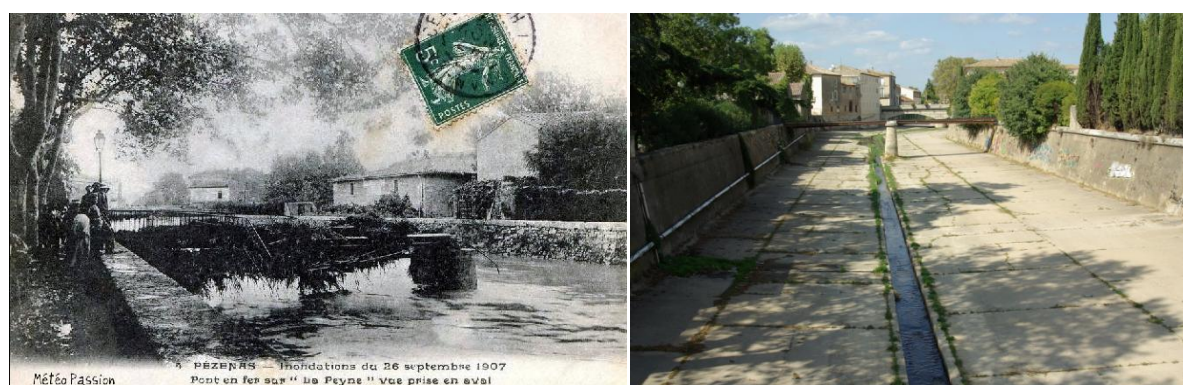
Figure 1.2: a) Pézenas bridge acting as a debris obstacle during the 1907 crues, (meteopassion, 2010) b) the concrete floodplain at Pézenas
