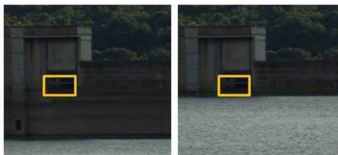
Figure 4.1: The water level before October 11 th 2009 and the expected (manipulated) water level on February 10 th 2010 relative to the 22m 3 /s spill (yellow cube).
