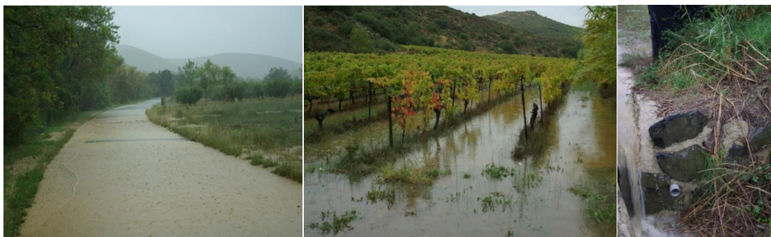
Figure XVI.2a-c: a) runoff from agricultural fields passing the road between Roujan and Vailhan (UTM x 524483,249 y 4821349,510) b) a flooded vineyard (UTM x 525030,671 y 4820712,005) c) runoff flowing from the flooded field into the stream with no water flowing out of the drain pipe
