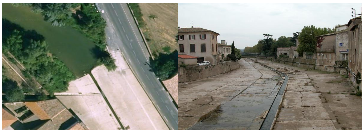
Figure 2.4: a) birds eye view of the narrow canalised river in Pézenas, b) front view of the canal
