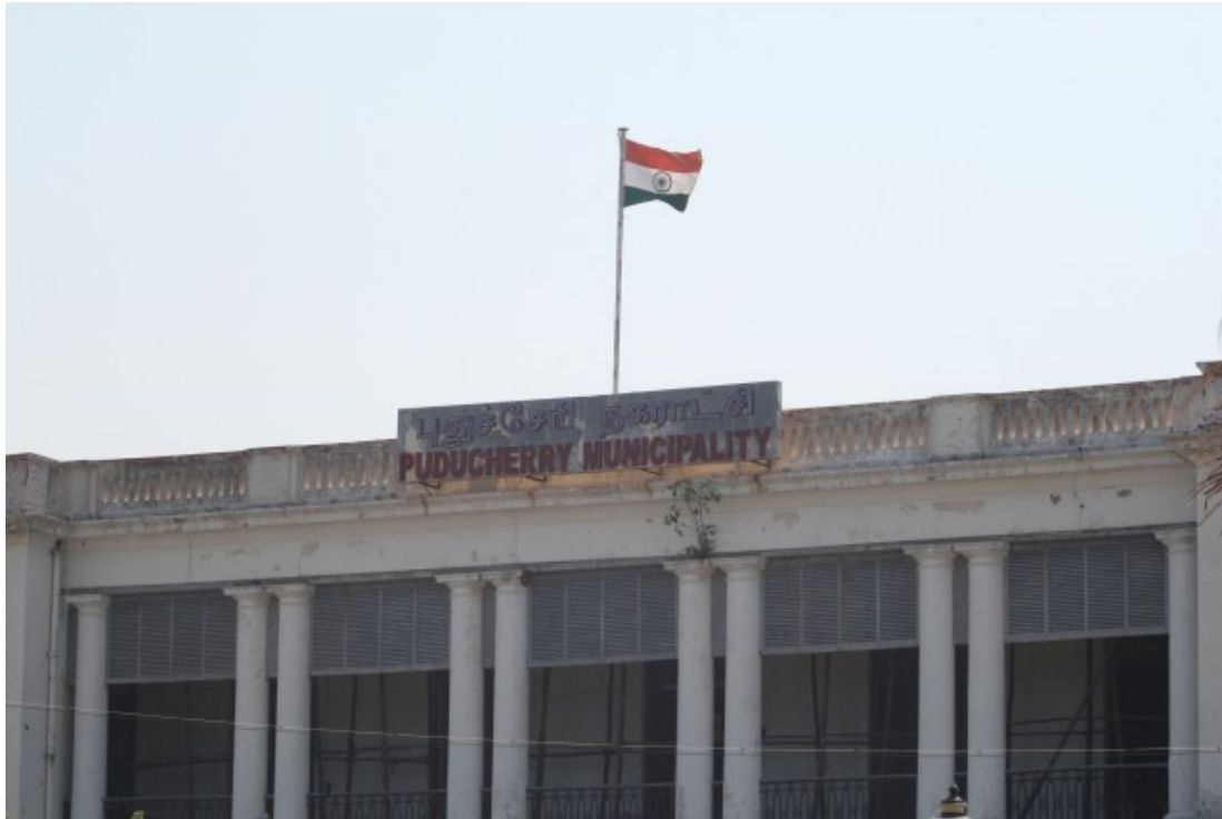
Image 1.5.10 Hotel de Ville (note the weeds growing out from the top of the middle pillars)
