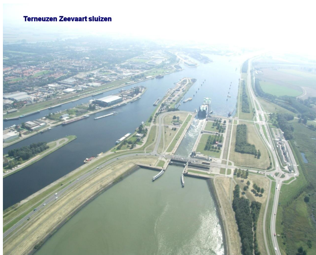
Figure 7.4: The entry to the Canal zone from the Western Scheldt: the sluice complex in Terneuzen
