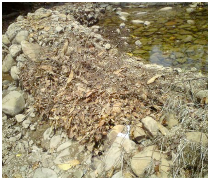
Figure 30: Retaining wall at the water source in Sital Tole
