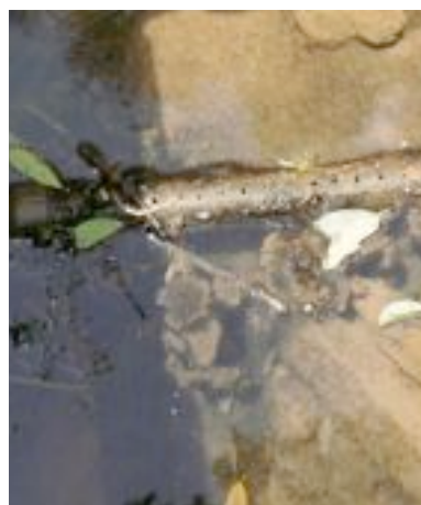
Figure 33: Intake at water source 2 surrounded by algae and organic waste
