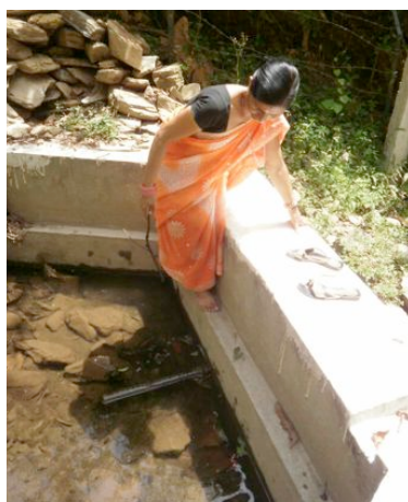
Figure 32: Water source 2 in Chintutar, serving 15 taps including school
