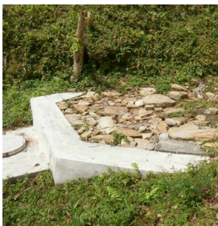
Figure 31: Water source 1 in Chintutar, serving 2 taps
