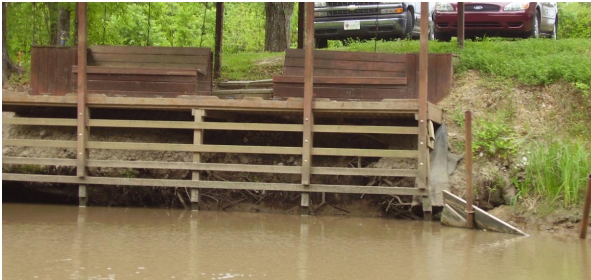
This wooden deck is at risk of caving in because of erosion. Photo taken by author.
