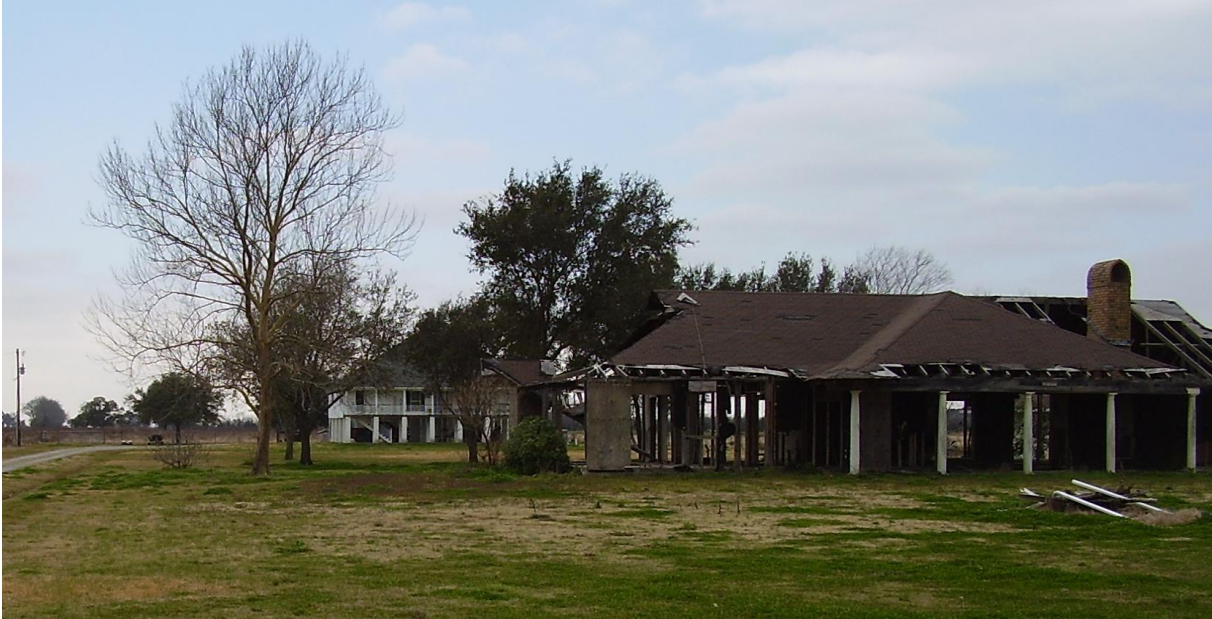
An elevated house is being built behind a damaged house. Photo taken by author
