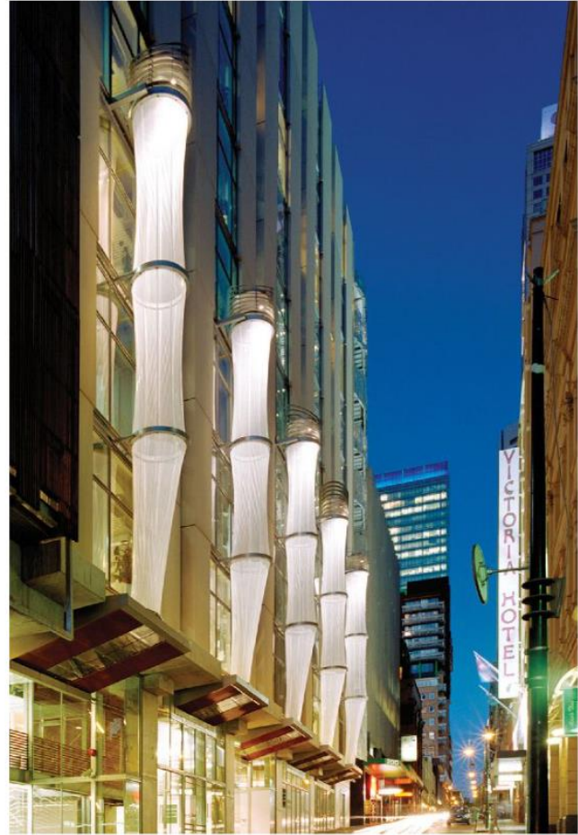
Figure 8 - The shower towers of CH2 capture air from their top side and condition it with water droplets to produce cool air for ventilating the interior spaces of the building. Figure retrieved from (Pearce, 2016a).
