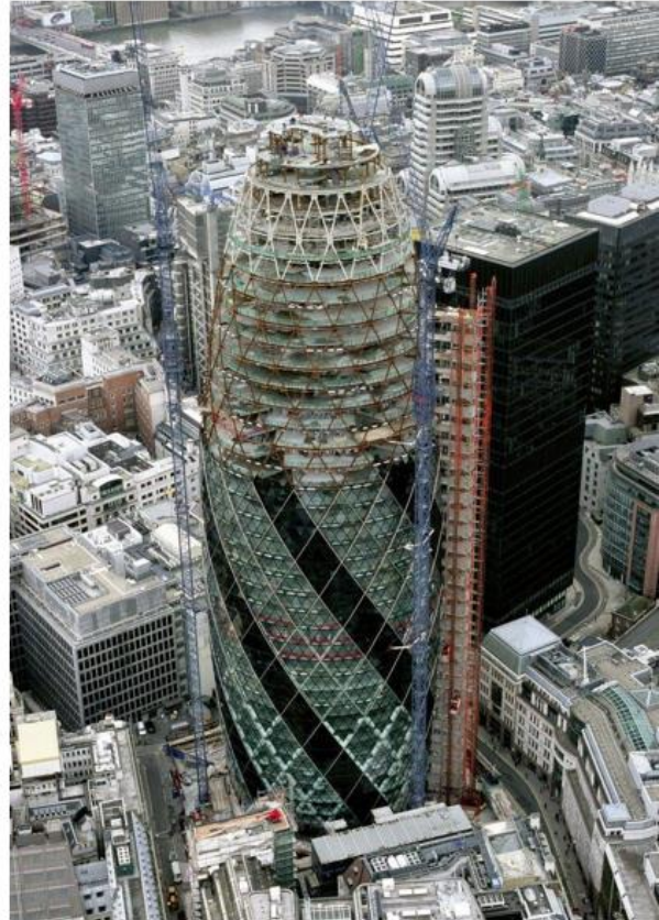
Figure 24 - The Gherkin tower's diagrid exoskeleton and façade enhance its wind resistance and make it significantly more material efficient than conventional moment-frame structures of its size. This exoskeleton is inspired by the Glass sponge, which successfully handles the strong deep-ocean currents using its lattice-like network of glass-like particles. Left image retrieved from (Moussavi, n.d.), and right image from (Dursin, 2023).
