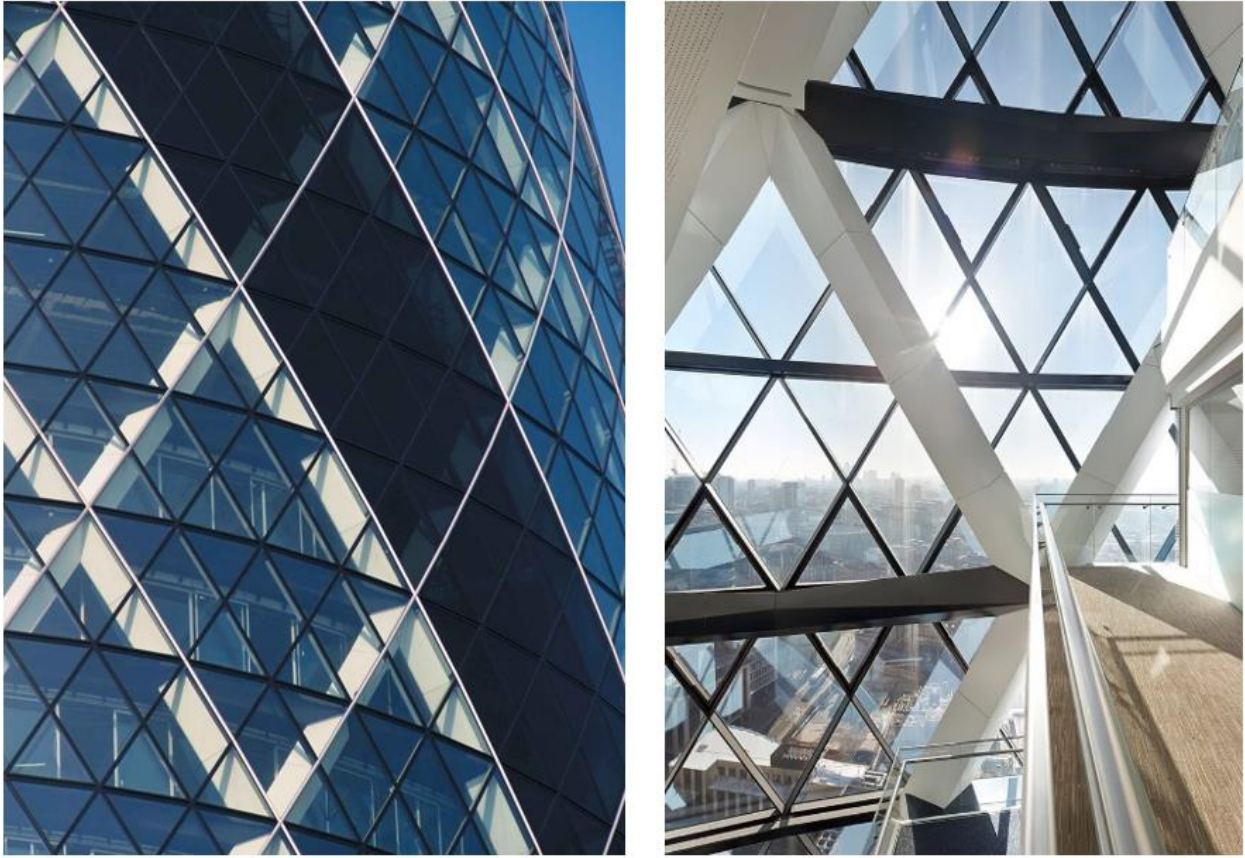
Figure 26 - Gherkin's light wells from exterior and interior angles. They bring in and disperse natural light to illuminate the circular floor plans. The darker line of glass consists of the blinds which are regulated based on the outdoor temperature and sunlight. For instance, if the outside temperature is between 20 and 26 °C, they open to allow ventilation. The detail of the steel diagrid structure is also visible. Left image retrieved from (Moussavi, n.d.), and right image from (The Gherkin, 2024).
