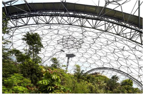
Figure 30 – A: Geodesic frames support the domes of the EP. B: The EP features two artificial enclosures that replicate natural biomes. One simulates a humid tropical rainforest with plants like banana trees, coffee, bamboo, and rubber; and the other represents a Mediterranean habitat, housing plants like olives and grape vines. Temperature and humidity levels are controlled to match each biome. Image A obtained from (The Eden Project, 2024) and B from (The Building Centre, 2021).
