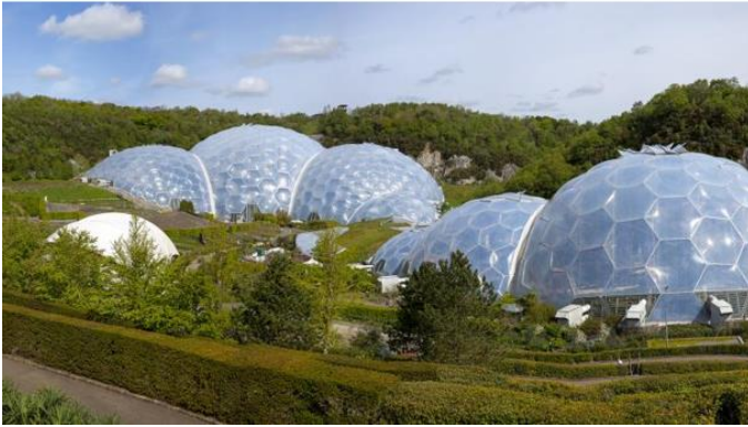
Figure 30 – A: Geodesic frames support the domes of the EP. B: The EP features two artificial enclosures that replicate natural biomes. One simulates a humid tropical rainforest with plants like banana trees, coffee, bamboo, and rubber; and the other represents a Mediterranean habitat, housing plants like olives and grape vines. Temperature and humidity levels are controlled to match each biome. Image A obtained from (The Eden Project, 2024) and B from (The Building Centre, 2021).
