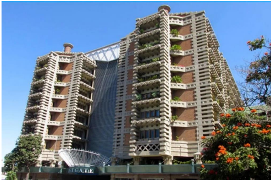
Figure 3 - EC building in Harare, Zimbabwe. The façade of the building is designed with deep balconies, and protruding stone and concrete shapes as and plants for heat dispersion and shading over the windows. EC's prickly or textured surfaces aren't efficient at collecting heat during the day, and they excel at emitting heat at night, thus cooling down the building for the next day. In contrast, smooth surfaces such as glass building envelopes would absorb more heat at night while radiating less back into space.
