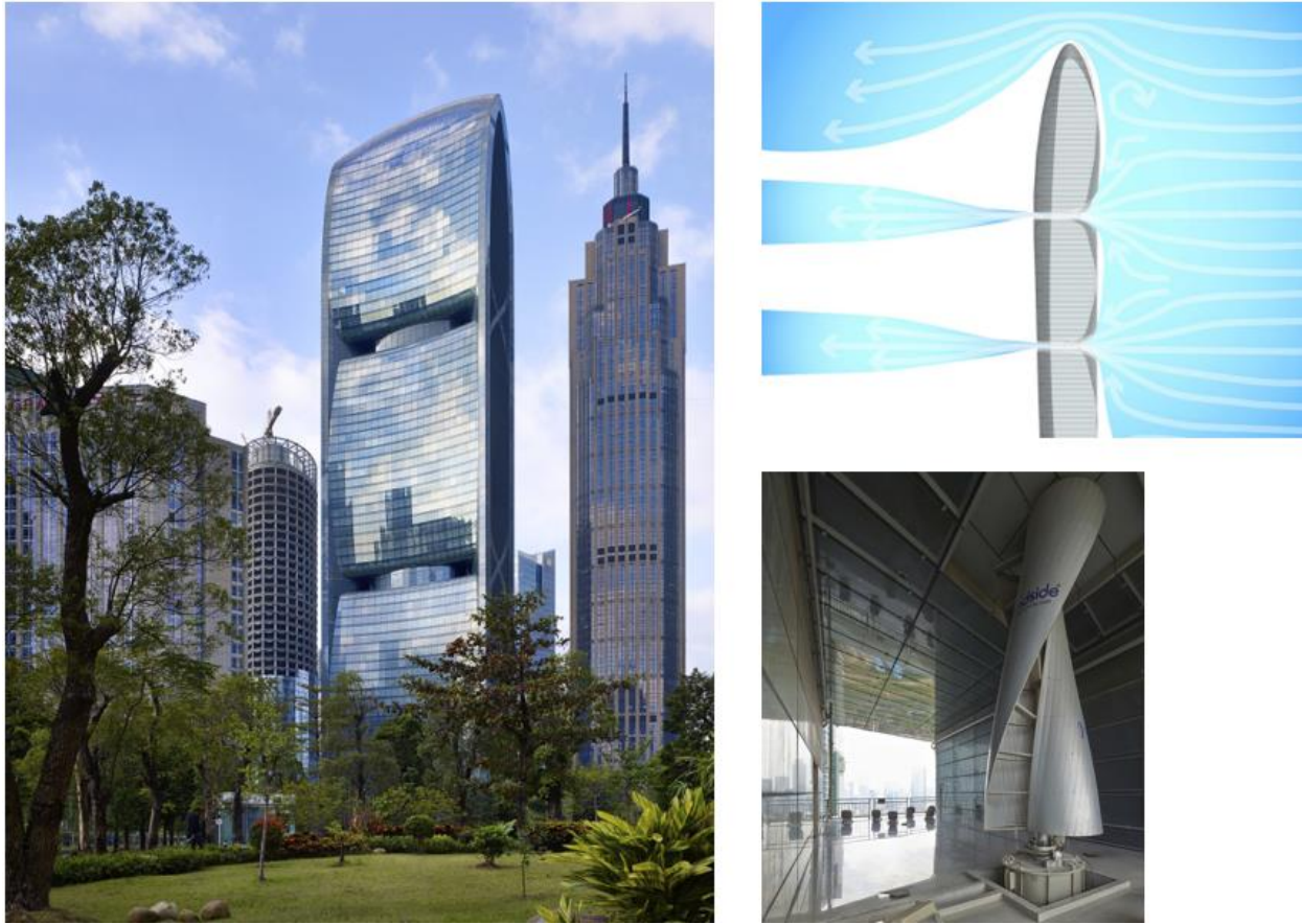
Figure 23 - Left: the design of the PRT in Guangzhou takes inspiration from sea sponges. Image obtained from (Council on Tall Buildings and Urban Habitat, 2024). Top right: the wind acceleration mechanism employed in the PRT (Gibson & Enns, 2020). The openings in the building suck in and accelerate winds to generate electricity using vertical axis wind turbines (bottom right – image from (Golenda, 2015)).
