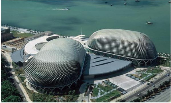
Figure 16 - The Esplanade's envelope inspired by the tropical Durian fruit. This envelope aims to limit the tropical solar radiation entering the building to prevent the building from overheating.
