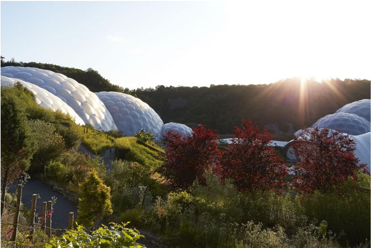
Figure 31 - The EP is located in a clay pit. The challenge of the project was to design buildings which could be sustained and adapted according to seasonal developments of the soil such as soil shrinkage. The designers overcame this challenge by opting for modular, lightweight domes made of replaceable ETFE pads, which are supported by geodesic structural frames which are also adaptable, lightweight, and modular. In practice, the ETFE is not a great acoustic insulator, and it can occasionally overheat the greenhouses during high temperatures as it lets in a lot of light. Additionally, while it is recyclable and its production comes with a lower impact than conventional glass and plastic, it is not biodegradable (Verbrugge et al., 2023; Wang, 2022). Image from (The Building Centre, 2021).
