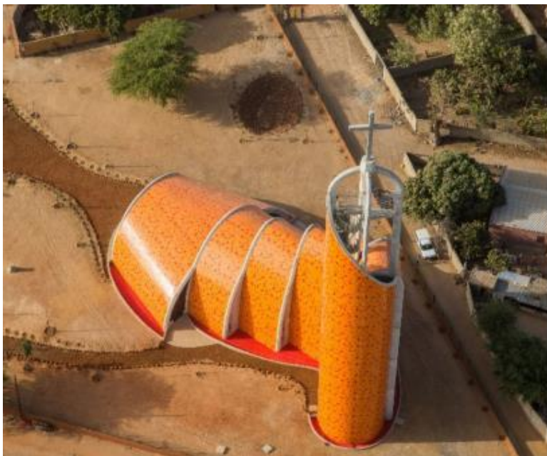
Figure 9 - The Nianing church's design resembles a spiral shell. Figure retrieved from (Blanco, Cruz, et al., 2021).
