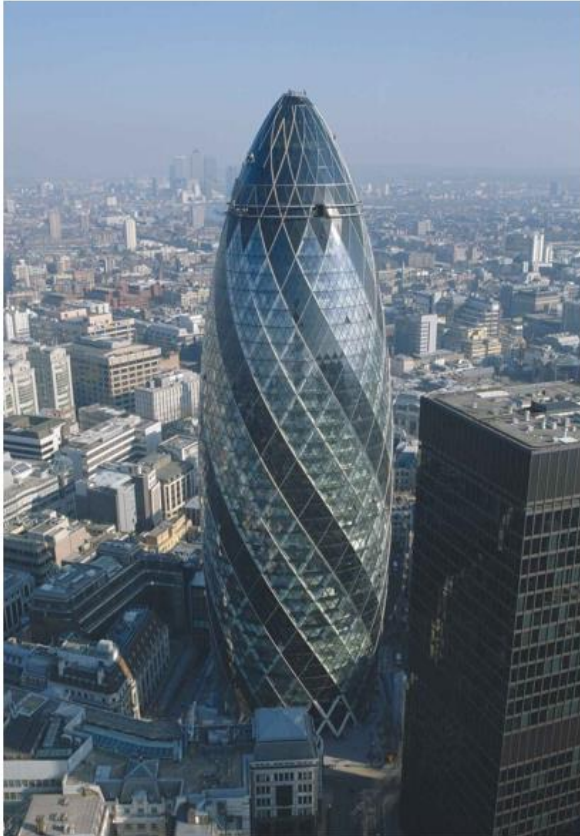
Figure 24 - The Gherkin tower's diagrid exoskeleton and façade enhance its wind resistance and make it significantly more material efficient than conventional moment-frame structures of its size. This exoskeleton is inspired by the Glass sponge, which successfully handles the strong deep-ocean currents using its lattice-like network of glass-like particles. Left image retrieved from (Moussavi, n.d.), and right image from (Dursin, 2023).
