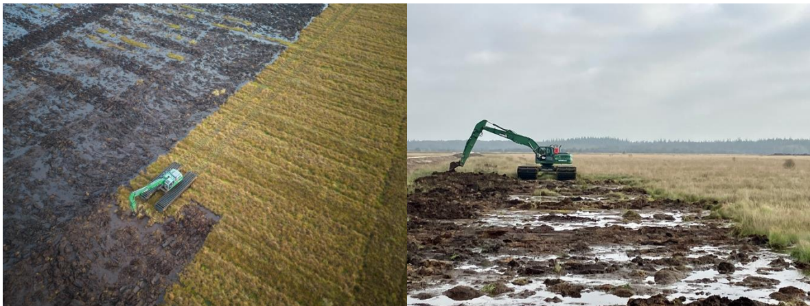
Fig 4. soil inversion taking place in site B in 2023, photos by: J, de Bruin, 2023
