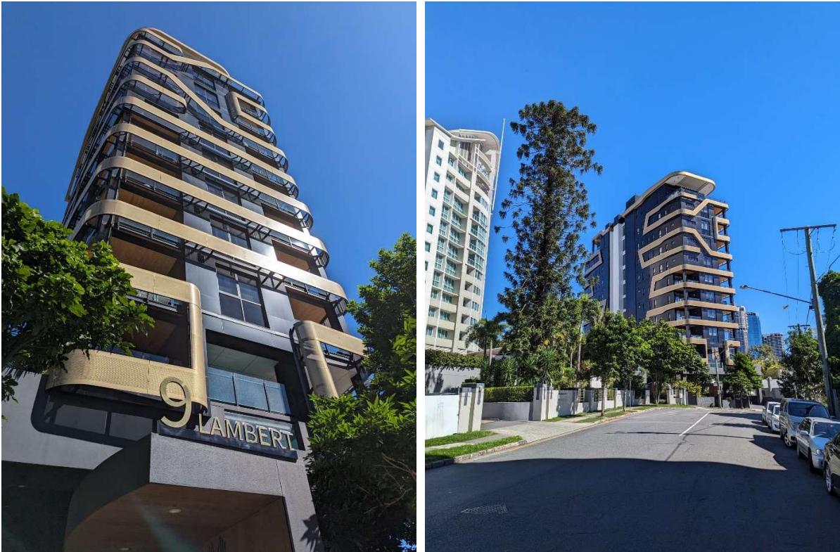
Figure 9: The Monterey – First CLT High-Rise Residential Building in Brisbane (Morgan, 2024)
