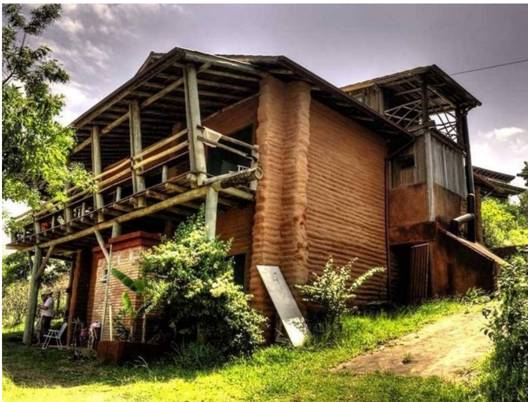
Figure 8 Casa Mae, a high standard, durable home, built using superAdobe sandbags.
