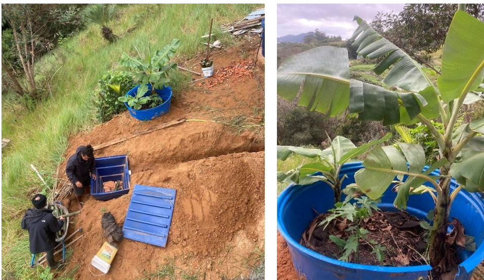
Figure 11 Grey water sanitation system using banana and papaya trees
