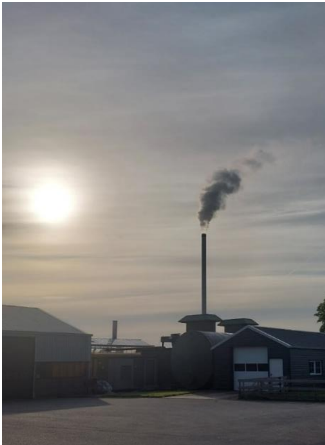
Figure 7 Combined Heat and Power Installation (CHPI)
