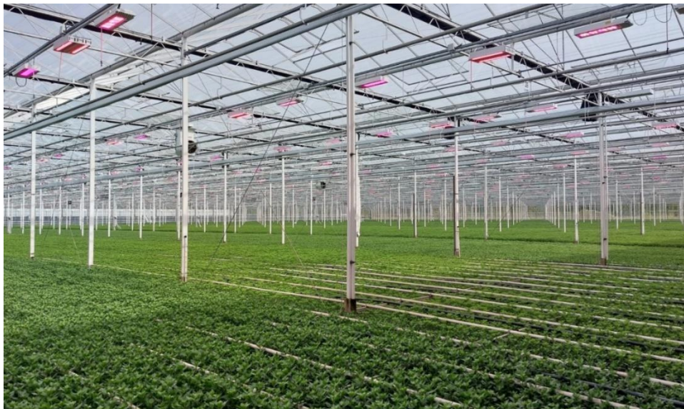
Figure 10 Large-scale greenhouse with artificial LED-lighting
