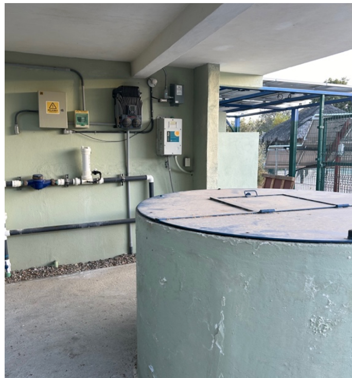
PHOTO 3: COVER OF THE WATER WELL AFTER RECONSTRUCTION
