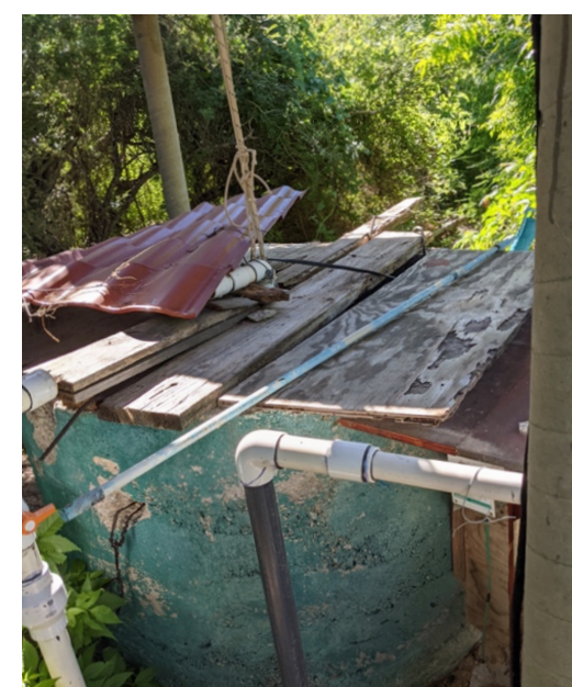
PHOTO 1: THE COVER OF THE WATER WELL BEFORE RECONSTRUCTION
