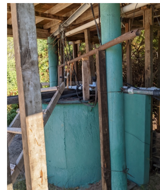
PHOTO 2: THE WATER WELL BEFORE RECONSTRUCTION
