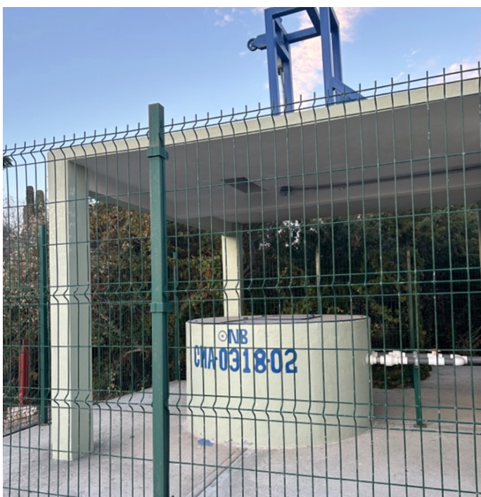
PHOTO 4: WATER WELL AFTER RECONSTRUCTION
