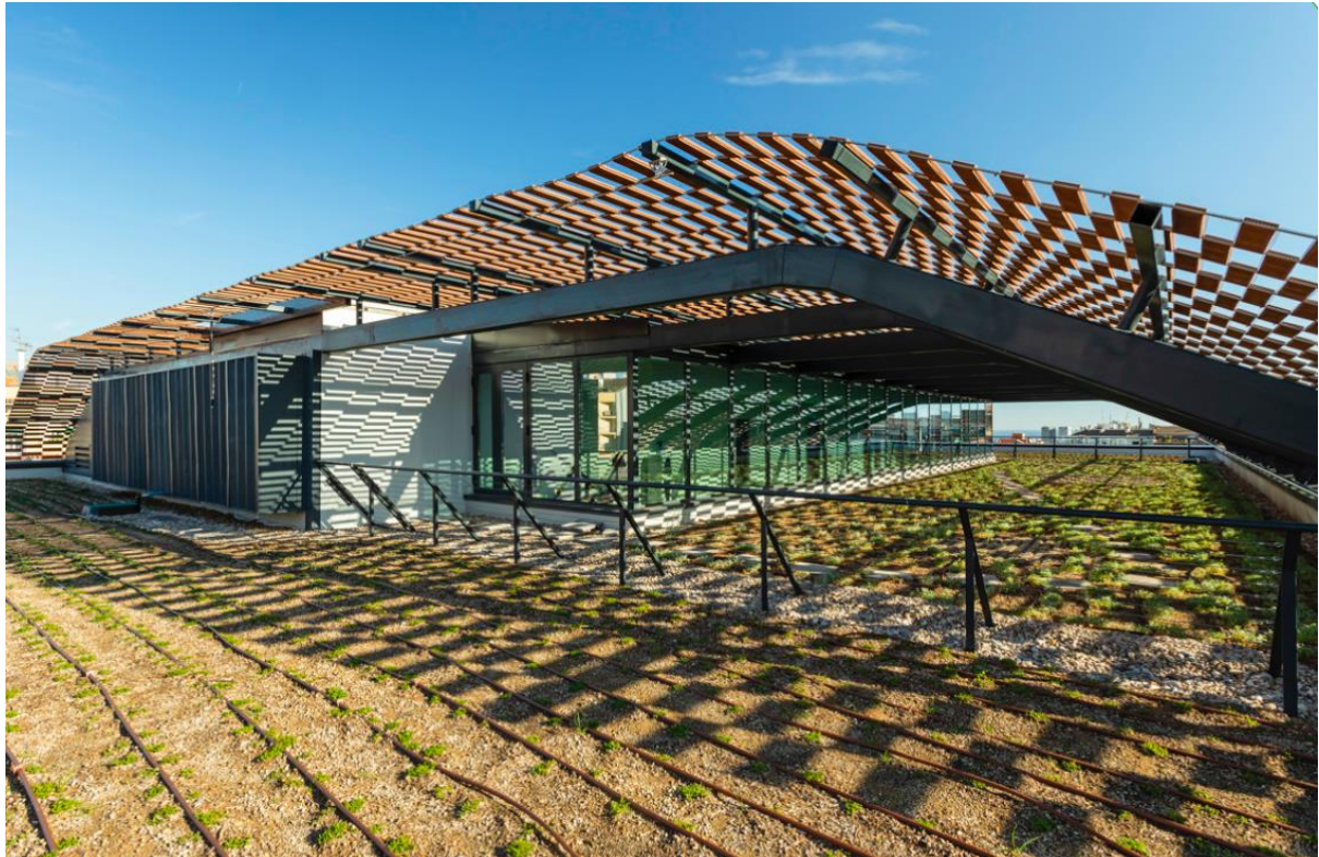
Image 20. Green roof winning project in Horta – First Contest 2017 Hospital Source: Ajuntament de Barcelona
