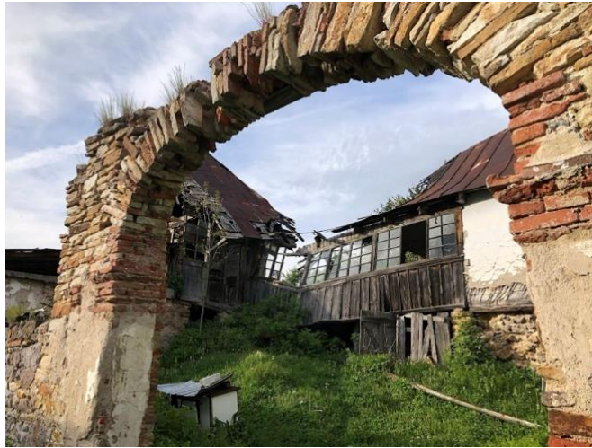
Figure 20 Abandoned house in Roșia Montană (personal archive, May 2024)
