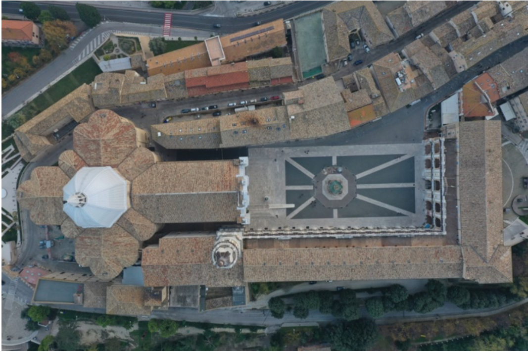
Figure 1.4. The sanctuary at Loreto seen from above.
