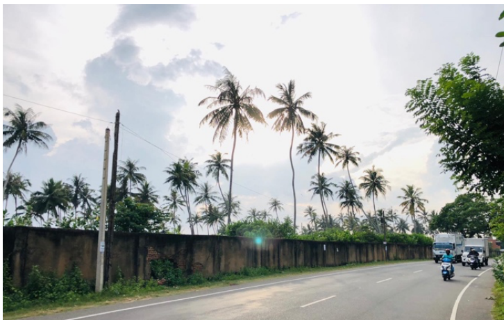
Figure 7. The wall blocking the beach view parallel to the Colombo Main Road, built by a private investor. Here, no coastal flood protection is present.
