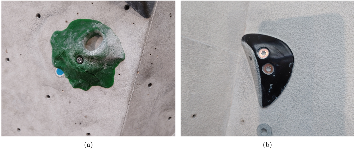
Figure 5.1: Examples of the two ways to secure a hold to the wall. Larger holds are attached to the wall using a bolt that goes through the centre of the hold as seen in Figure (a). Smaller holds do not have the space for this bolt and as such are attached to the wall using several screws driven directly through the plywood walls as seen in Figure (b).
