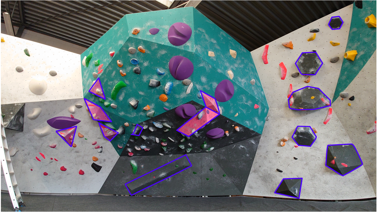
Figure 3.1: An example of an indoor bouldering wall. The coloured walls are made out of plywood sheets which are attached to a metal scaffolding at the back to create structure. Different coloured holds are attached to these walls. Each set of coloured holds defines a different route up the wall. The purple outlined volumes augment the walls and add new ways to create a route.
