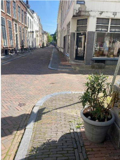
Figure 29 Crossing in Herenstraat
