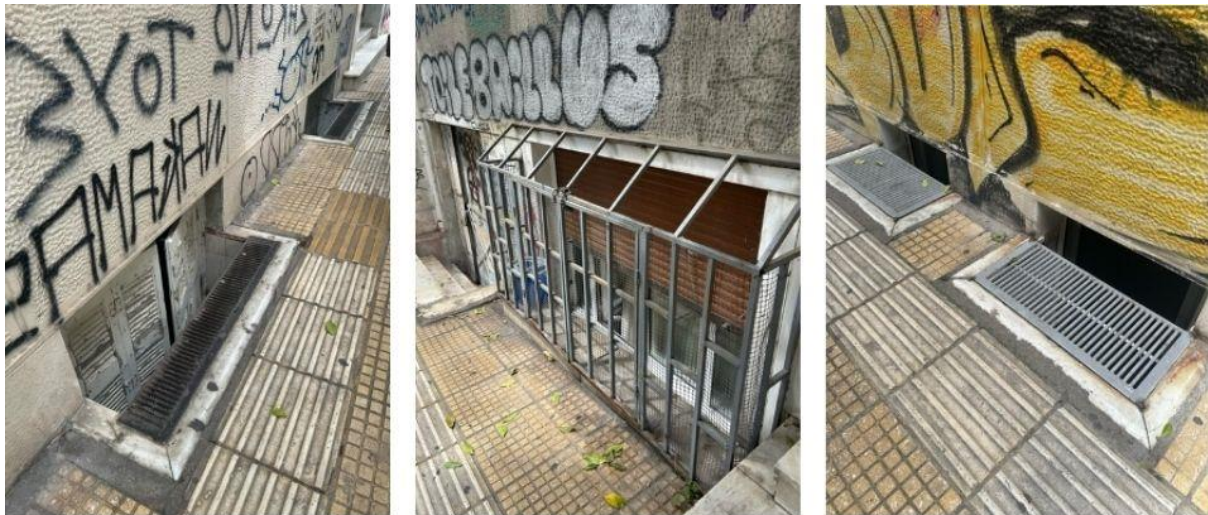
Figures 6, 7 & 8: Basement apartments as seen from the sidewalk
