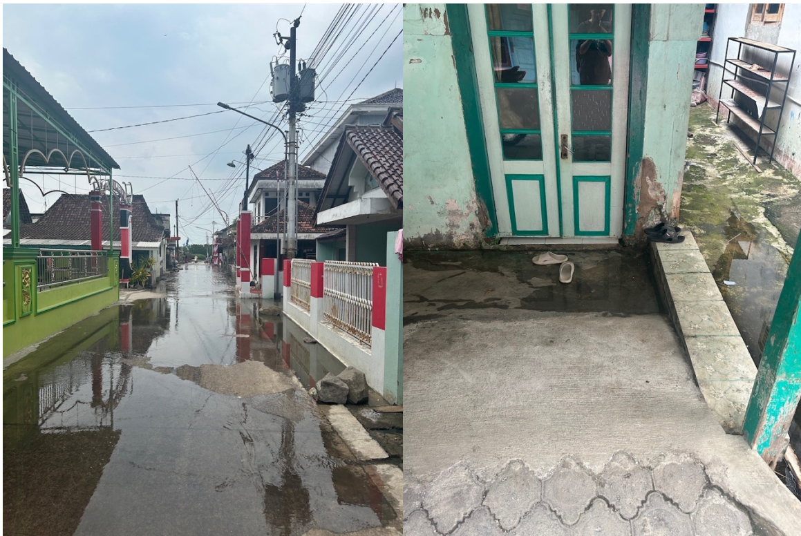
Coastal inundation in Mangkang Wetan. Source: personal archive (April 2024)
