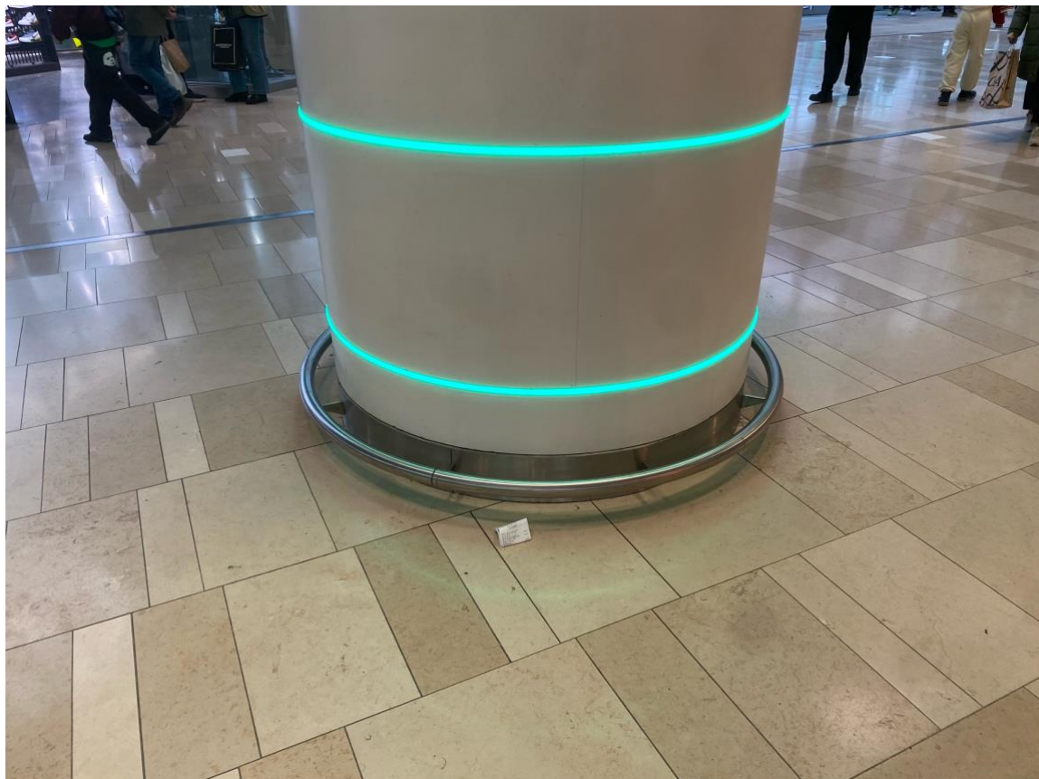
Photograph VII: Steel tube around a column that discourages people from sitting against it (own data).
