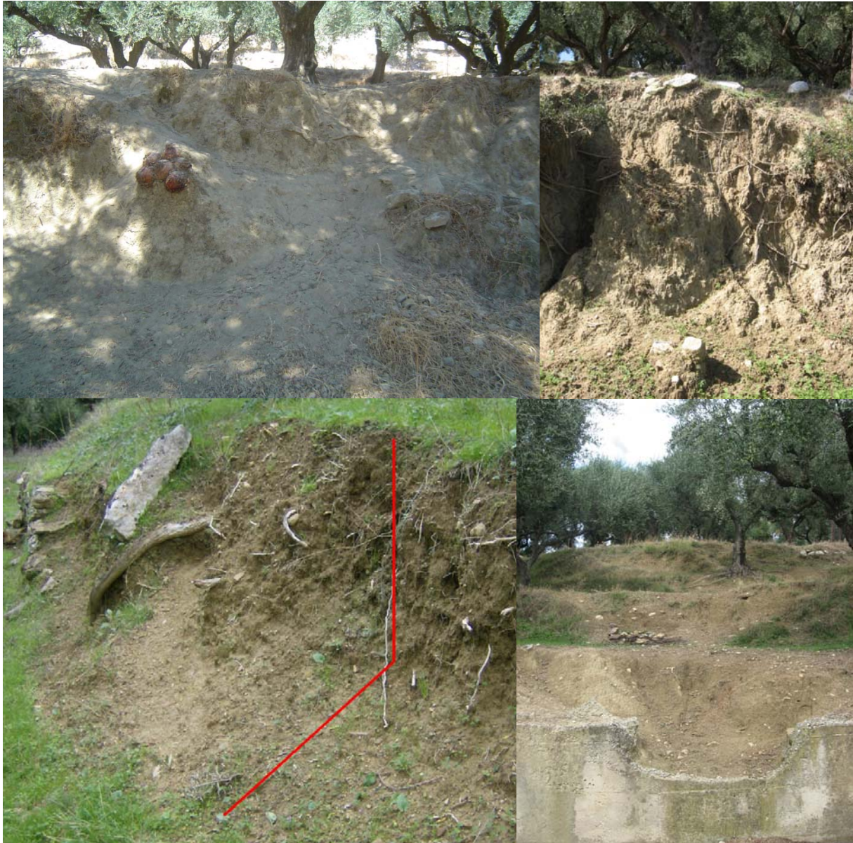
Figure 12: Top left: Erosion/deposition (485717, 4172184). Top Right: Erosion/deposition below the road (485702, 4172221). The pictures on top are from August 2009.
