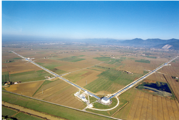
(b) An aerial photo of the Virgo detector in Italy. This interferometer has an arm length of 3 km, which is further extended by light storage arms. Picture from [65].
