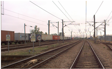
Figure 5: Cropped video frame of a part of the track. On the left the two wayside objects with exclamation marks are clearly visible, without objects obstructing the laser scanner.
