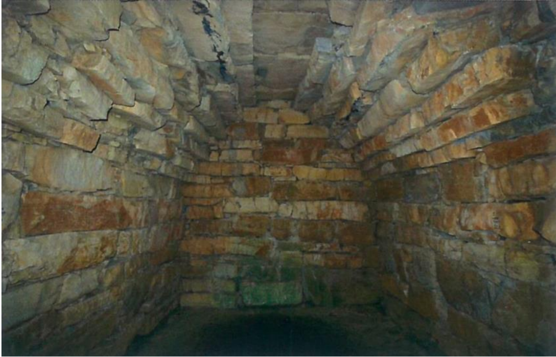
Figure 21: Interior of the main chamber of the north hypogeum at Montecalvario, with corbeled vaulting.
