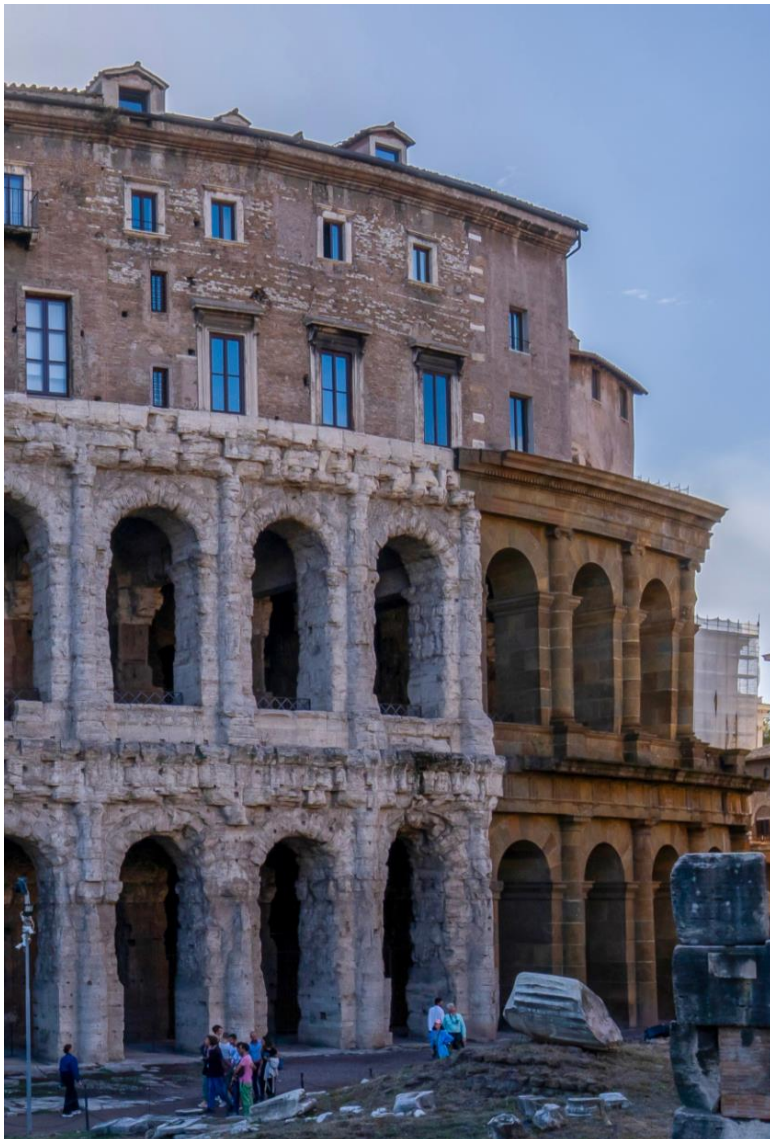
Figure 31: The Temple of Marcellus, with Doric columns and entablature at the lower level, 13 BC, Rome.
