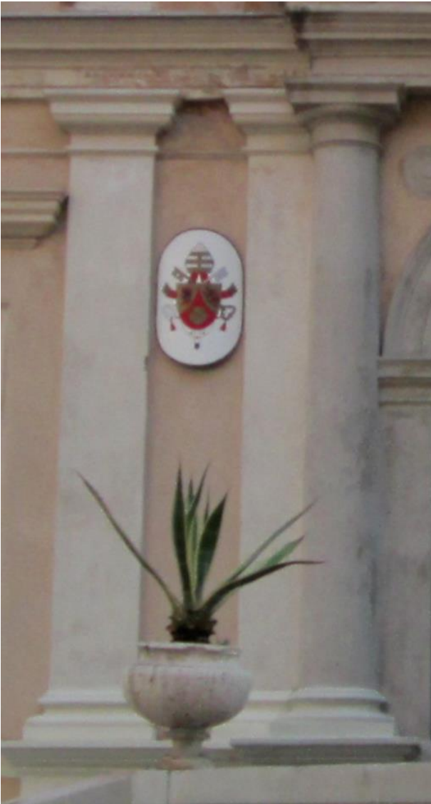
Figure 59: Giulio Romano, detail of the façade of the Villa Lante, Tuscan columns, unfluted and with Attic bases, Janiculum, Rome.
