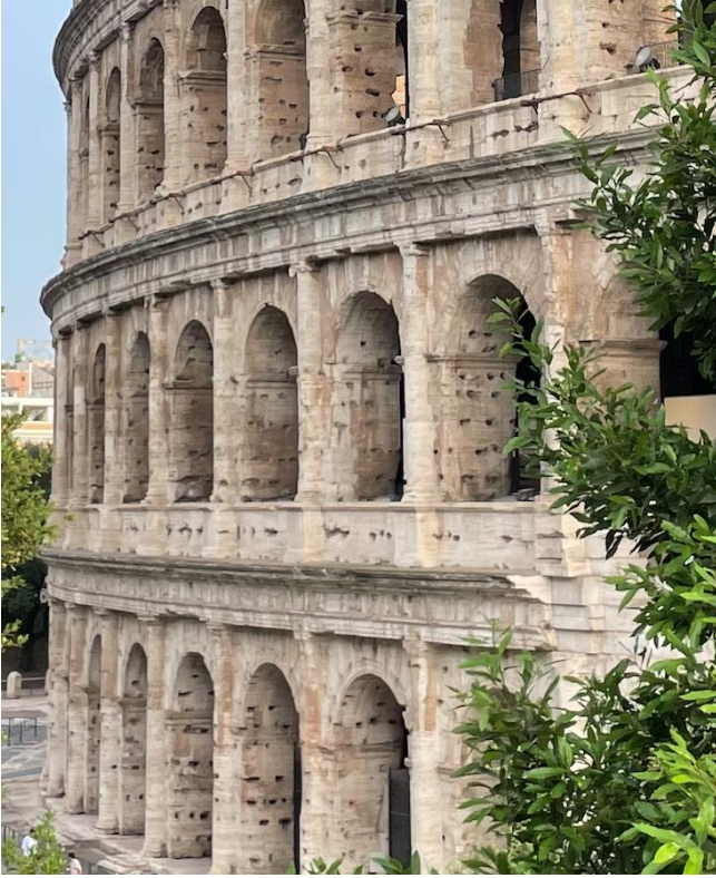
Figure 32: The superimposed orders of the Colosseum, with Doric at the lowest level, AD 70-80, Rome.
