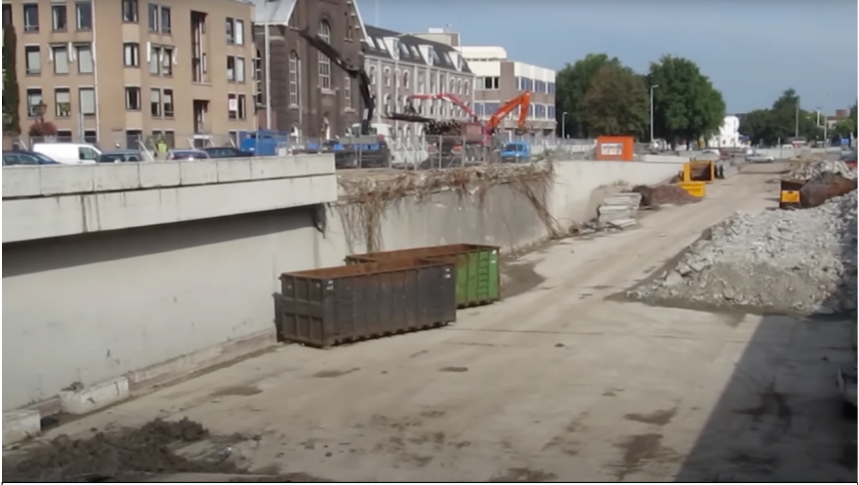
Image 6: Demolition of the Catharijnabaan in 2009. Source: YouTube
