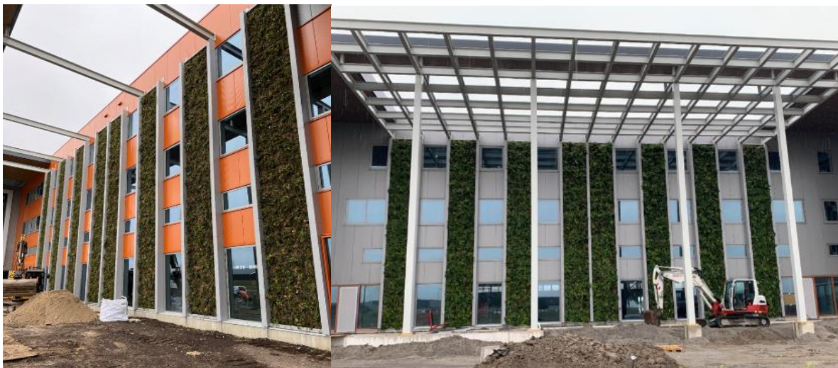
Living Walls Hoofddorp left: HAO-LW, right: HAG-LW (under construction)
