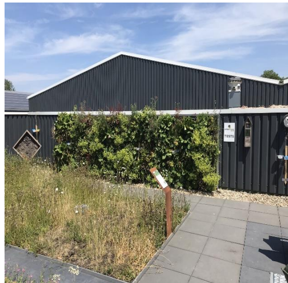
Living Wall Odijk: OSL-LW
