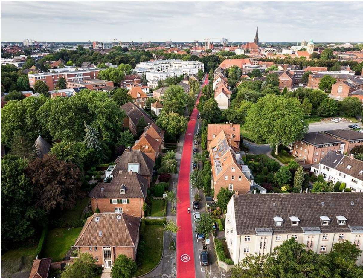
Figure 1: View Goldstraße (Schulte, 2020)
