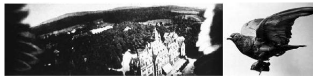
Figure 2: One of the pigeons of the Bavarian Pigeon Corps with the mounted camera, shooting areal photos Source: Remote Sensing tutorial Overview, n.d.
