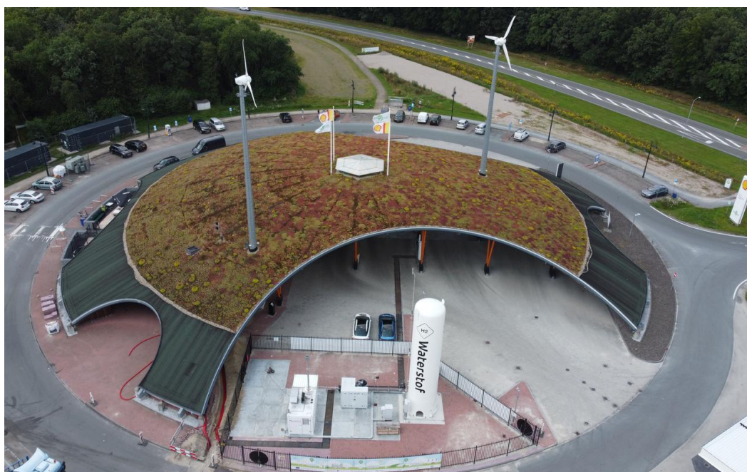
Fig. 4. A clean energy hub for road transport
