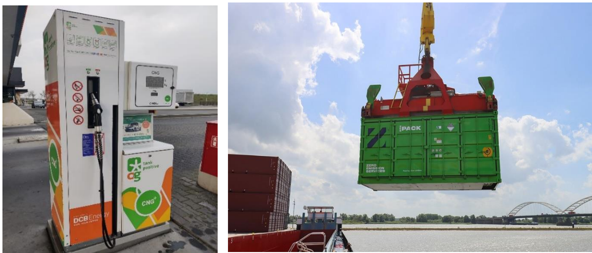
Fig. 5: Left: fuelling point for road transport (BIO CNG), Right: fuelling point for water transport (electric battery container)
