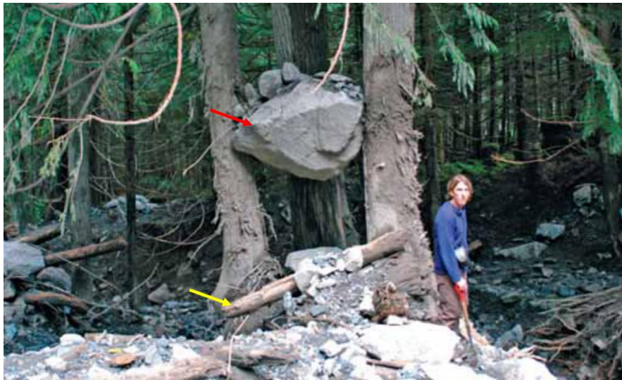
Figure 19 Example of obstruction formation in a real forest. The yellow arrow indicates an obstruction formed due to a captured log with gravel captured upstream of the log. The red arrow shows a captured rock. The rock was transported in the debris flow and according to Wilford et al., (2005) provides an indication of the debris flow depth. Adaption of figure 11 from Wilford et al., (2005).
