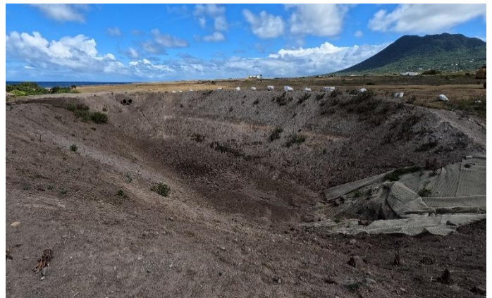
Figure 6.5: Large infiltration basin created inside a gully. Erosion by inflowing water is controlled with a geotextile. A spillway is installed in the dam at the downstream end of the basin. This photo is included in APPENDIX 4
