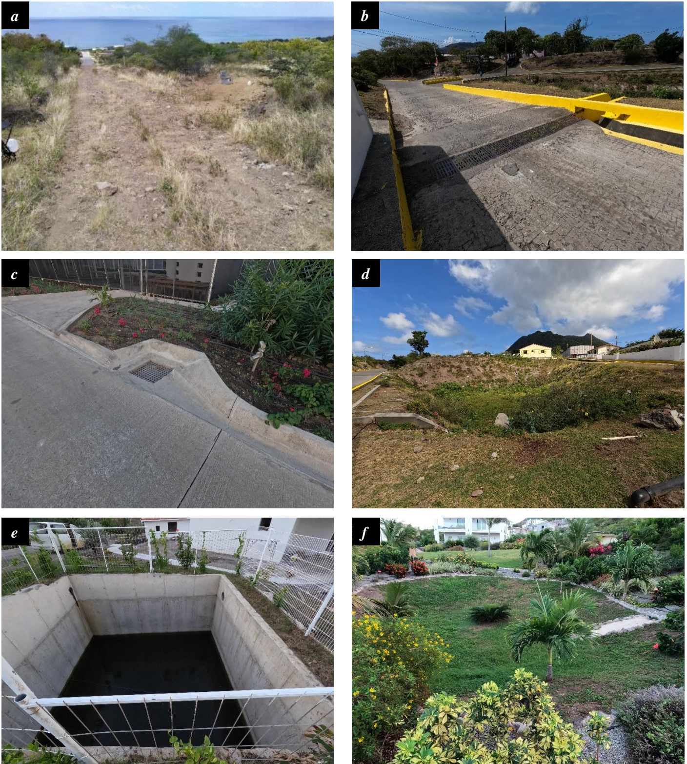
Figure 6.1: Some existing water management applications on Sint Eustatius. a. Infiltration pit at the side of an unpaved road; b. A linear drain followed by a speed bump. It discharges directly into an infiltration basin; c. A roadside storm drain; d. Large infiltration basin; e. Runoff storage facility; f. Small bioswale / infiltration basin. These photos are also included in APPENDIX 4 .
