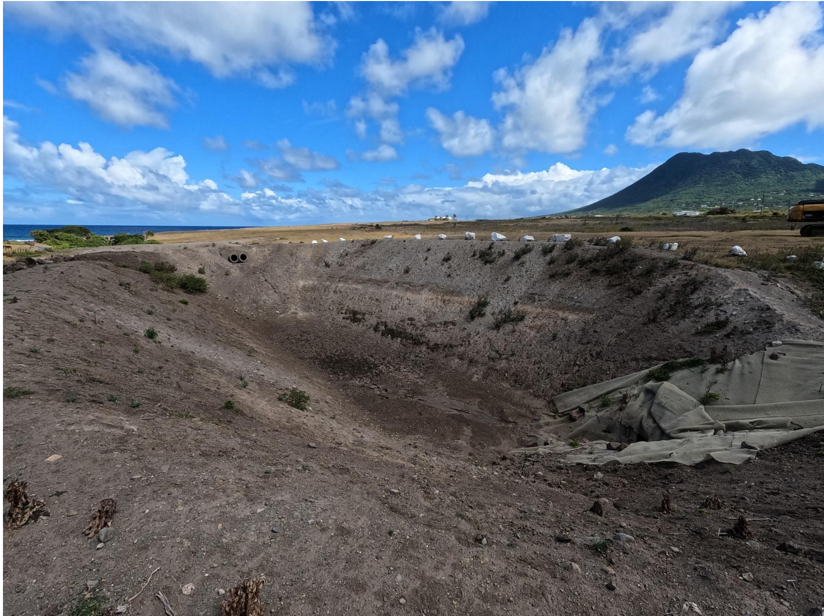
Photo 7 – Large infiltration basin created inside a gully
