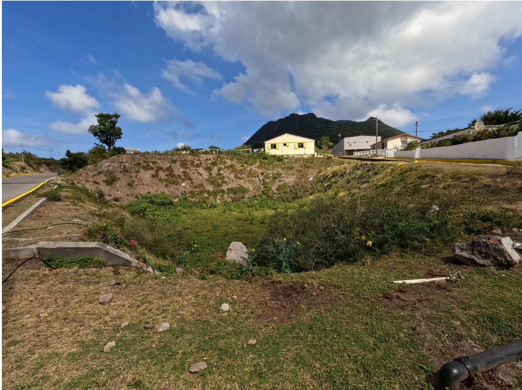
Photo 4 – Large infiltration basin
