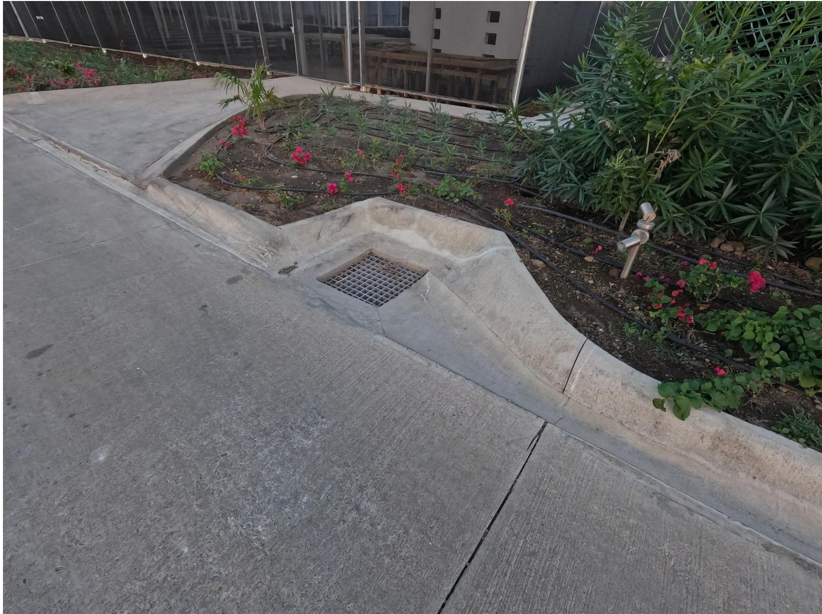
Photo 3 – Roadside storm drain
